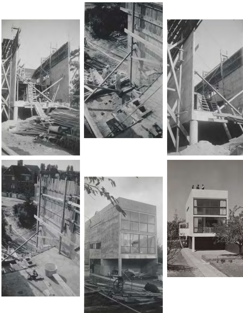
[Fig. 7-12] Images documenting the construction process of the house Anchersvej 6. Source: Royal Danish Library.
