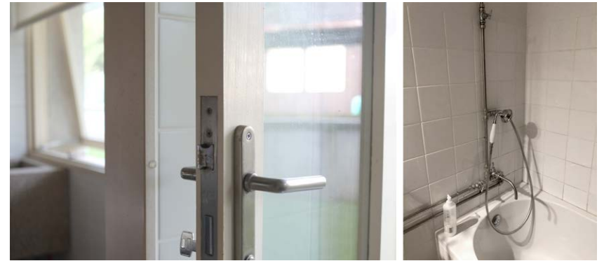
[Fig. 9] New residents maintain Siza's 'micro-technologies' in the flat, such as door levers and the window system (Left). In the bathroom, parts and external pipes are not original but were chosen by new owner-architects to match the original concept (Right). Photos: Author 1, 2023.
