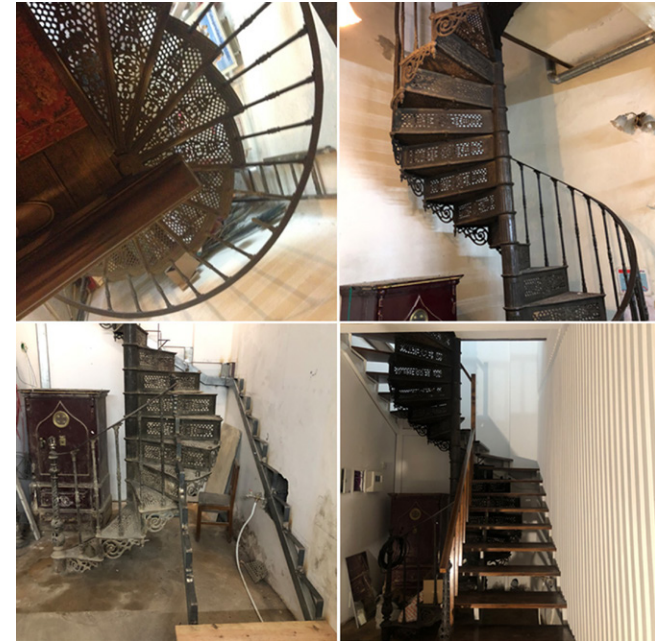
[Fig.9] Spiral cast-iron staircase and new overlapping staircase. © Authors, 2020.
