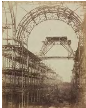
[Fig.5] Construction of the Grand Palais, Paris, photograph by A. Chevojon, 1897–1900. Le Grand Œuvre , Photopoche.
